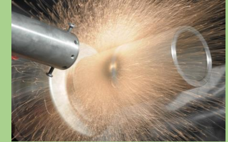
Reparation of a crack
